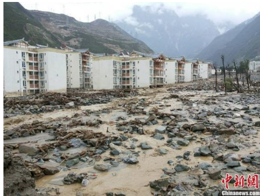
Reconstruction site was affected
