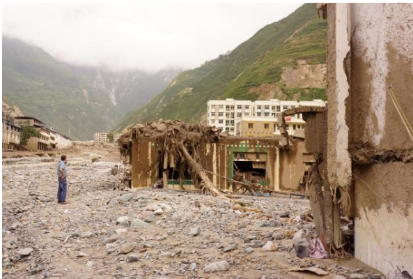
Destroyed houses near the outlet
