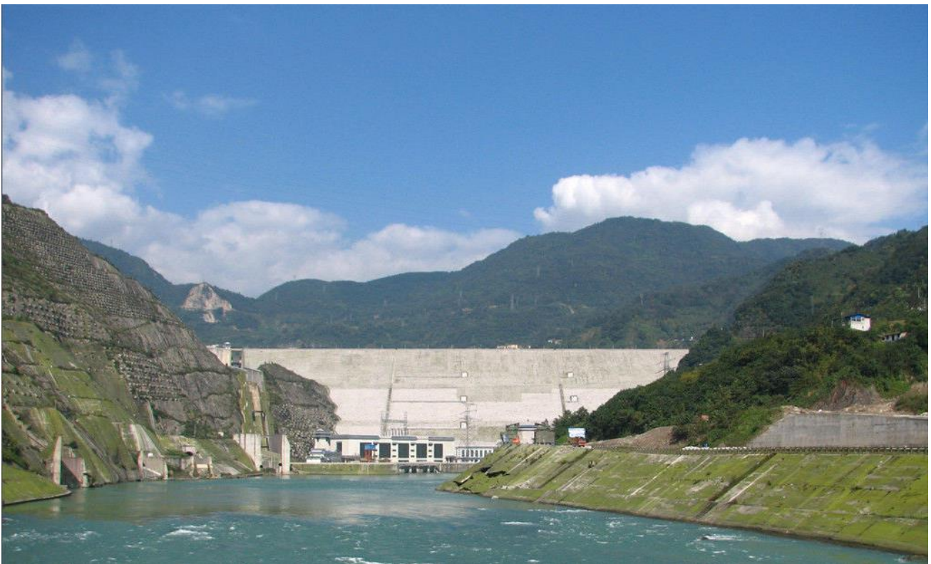
Zipingpu dam and hydro-power station
