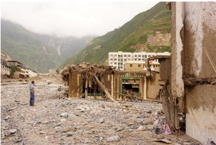
Destroyed houses near the outlet
