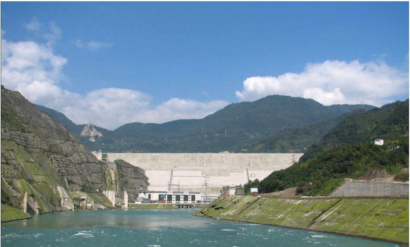
Zipingpu dam and hydro-power station
